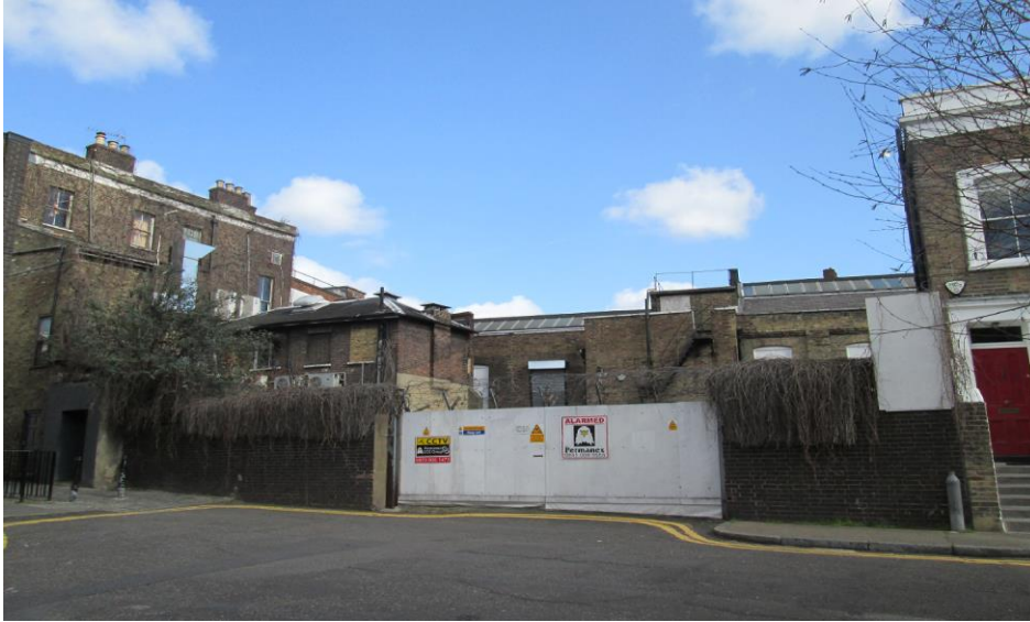
Photograph 5: The Queens Head Street entrance to the site
